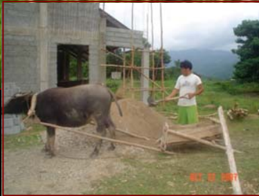
They are hauling the gravel and sand by using caribou and cart.
