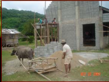
They are hauling the gravel and sand by using caribou and cart.
