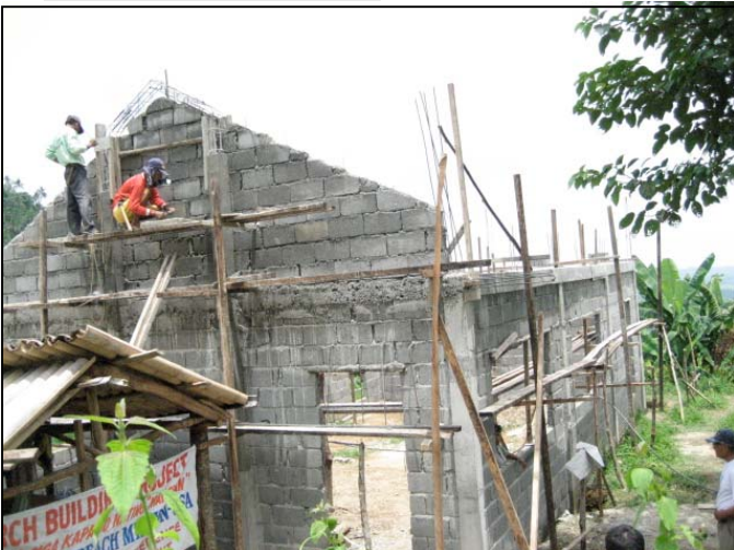
Working on Church
